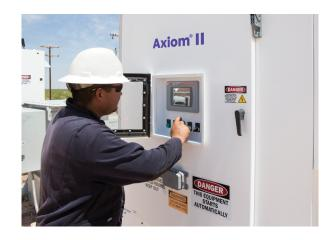
Running on a high-speed processor in the Axiom II drive, the vector control algorithm is able to resolve the applied three-phase stator current into two components: a magnetizing current and a torqueing current. Adding specific downhole motor characteristics as input, the algorithm permits independent control and adjustment of the two quantities.
