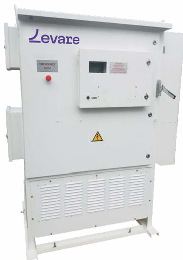
The Model-15 VSD controller is further equipped with additional advanced software that supports drive performance in response to challenging well conditions such as gas and solids. Specialized algorithms are available to the operator that help the downhole pump system overcome conditions such as gas lock, scale buildup, or difficulty at startup.
